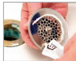
...or installs with silicone (if drain crossbars are missing)
